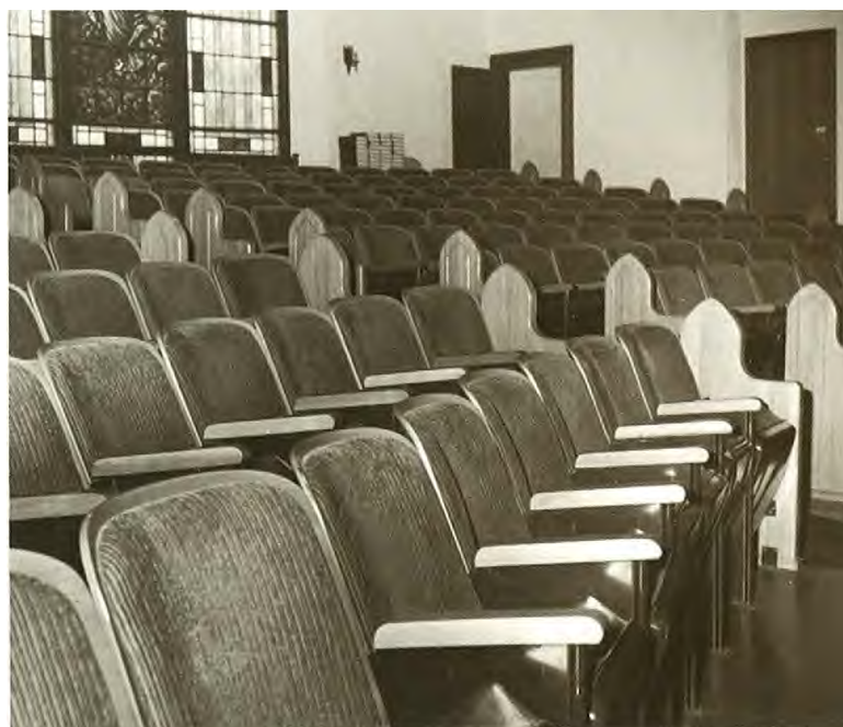
Balcony chairs installed, 1980
