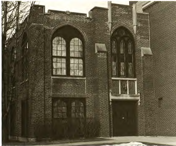
Sunday school addition, 1929
